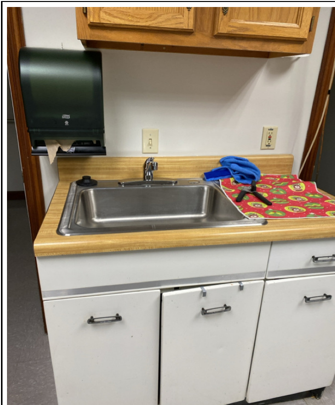
2/7/2024 - 318-1 - Admin Building - Kitchen
